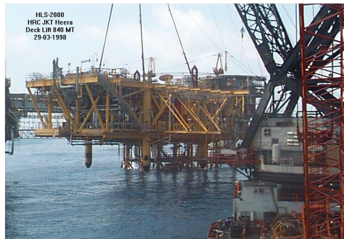
Deck Being Installed offshore using a derrick mounted heavy lift crane.
