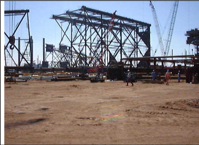
Jacket under fabrication at yard.
